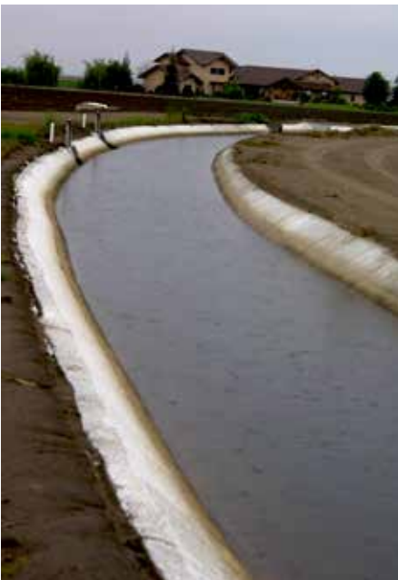
THE PROJECT ALSO STRAIGHTENED SEVERAL MEANDERING SEGMENTS OF THE DITCH TO IMPROVE DELIVERY TIME TO THE FARM.
