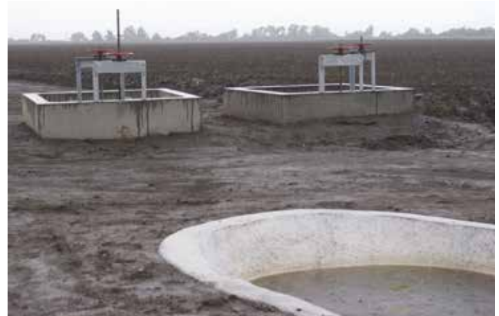
NEW WASHOUT DRAINS HAVE ELIMINATED MESSY WASHOUTS ON THE GAMBONI DITCH AND HELPED CLEAN UP FIELDS.
