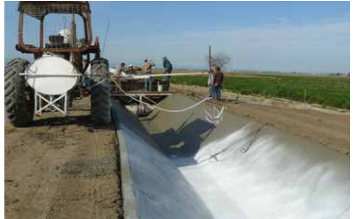
WORK ON THE SILO DITCH COMMUNITY DITCH IMPROVEMENT PROJECT INCLUDED REPLACING EARTHEN DITCH WITH MORE THAN TWO MILES OF CONCRETE LINING AND PIPELINE.
